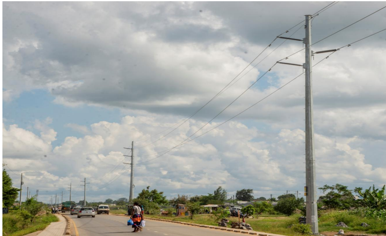
Construction of 132kV Single Circuit Transmission Line from Coventry – Waterworks, Coventry – Jimmy – Chawama for ZESCO in Lusaka
