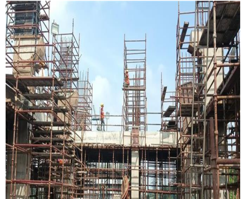
Data Center substation & line - construction of 220/33 KV GIS Substation and associated Transmission line Substation: 1 (no.) Status: On-going
